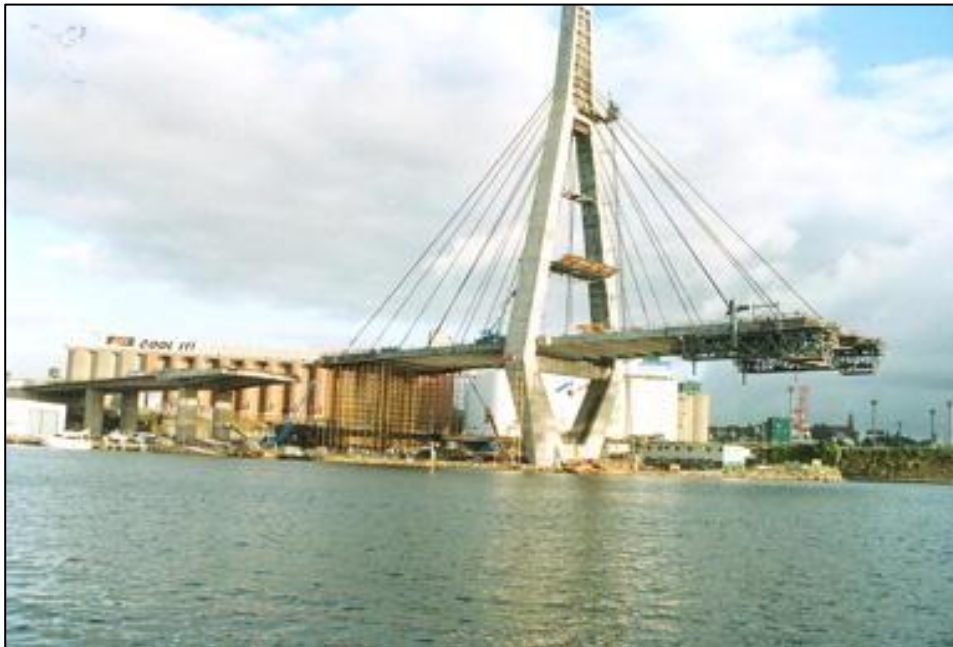
Figure 7: The Anzac Bridge under construction, the c.1975 Silos are in the background.
