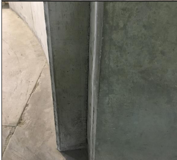
Figure 25: The 300mm thick reinforced concrete ring.
